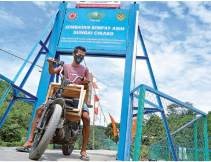
Tzu Chi worked with the military, villagers, and volunteers from Vertical Rescue Indonesia to rebuild a bridge in Depok, Garut, Indonesia. The new bridge was inaugurated on January 6, 2021. MOCH GALVAN
