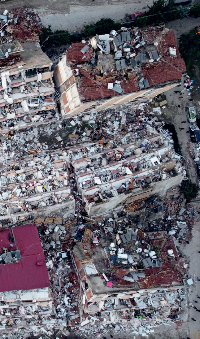
A bird's eye view of a central area in Hatay Province, southern Türkiye, after the quakes. Almost all the local buildings have collapsed. COURTESY OF TPG IMAGES
