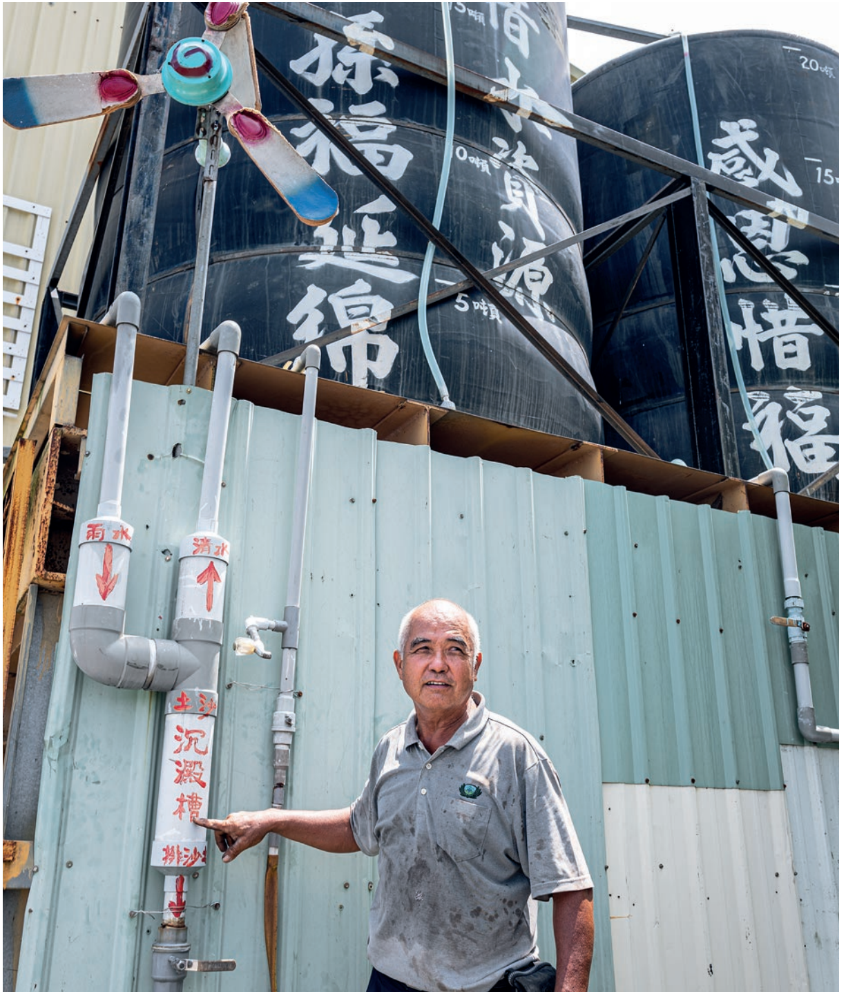
Lin Jin-guo, a volunteer at the Tzu Chi Nanpu Recycling Station in central Taiwan, designed a rainwater harvesting system using recycled water tanks of various sizes. The collected rainwater is filtered and used within the station, significantly reducing tap water consumption.
